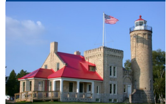
Mackinac Point Lighthouse
